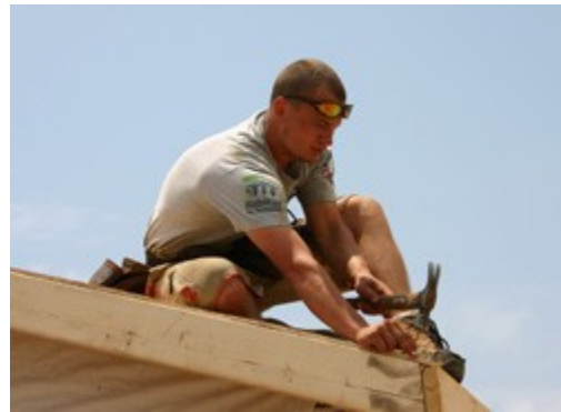
Habitat AmeriCorps member building in the Mississippi Gulf Coast.
