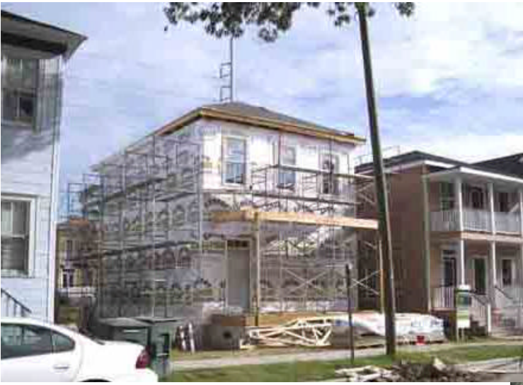
Mid-October front view shows the Tyvek barrier in place and the beginnings of a full roof over the front porch.
